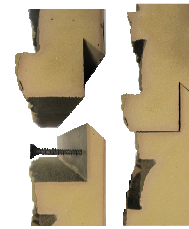
Tongue and groove top-to-bottom interlock.
