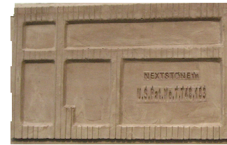
Recessed panel back and weep channels.
