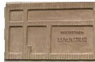
Recessed panel back and weep channels.
