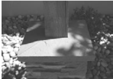
2 Piece Cap Installed
