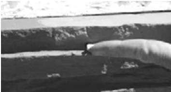
Apply Caulk to Screw head
