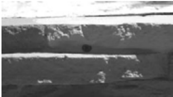
Exposed Screw Head
